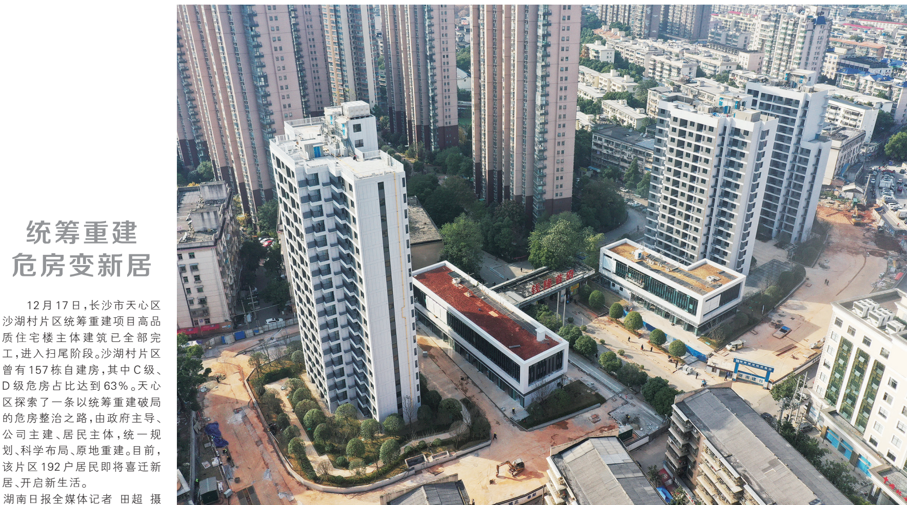
统筹重建 危房变新居
